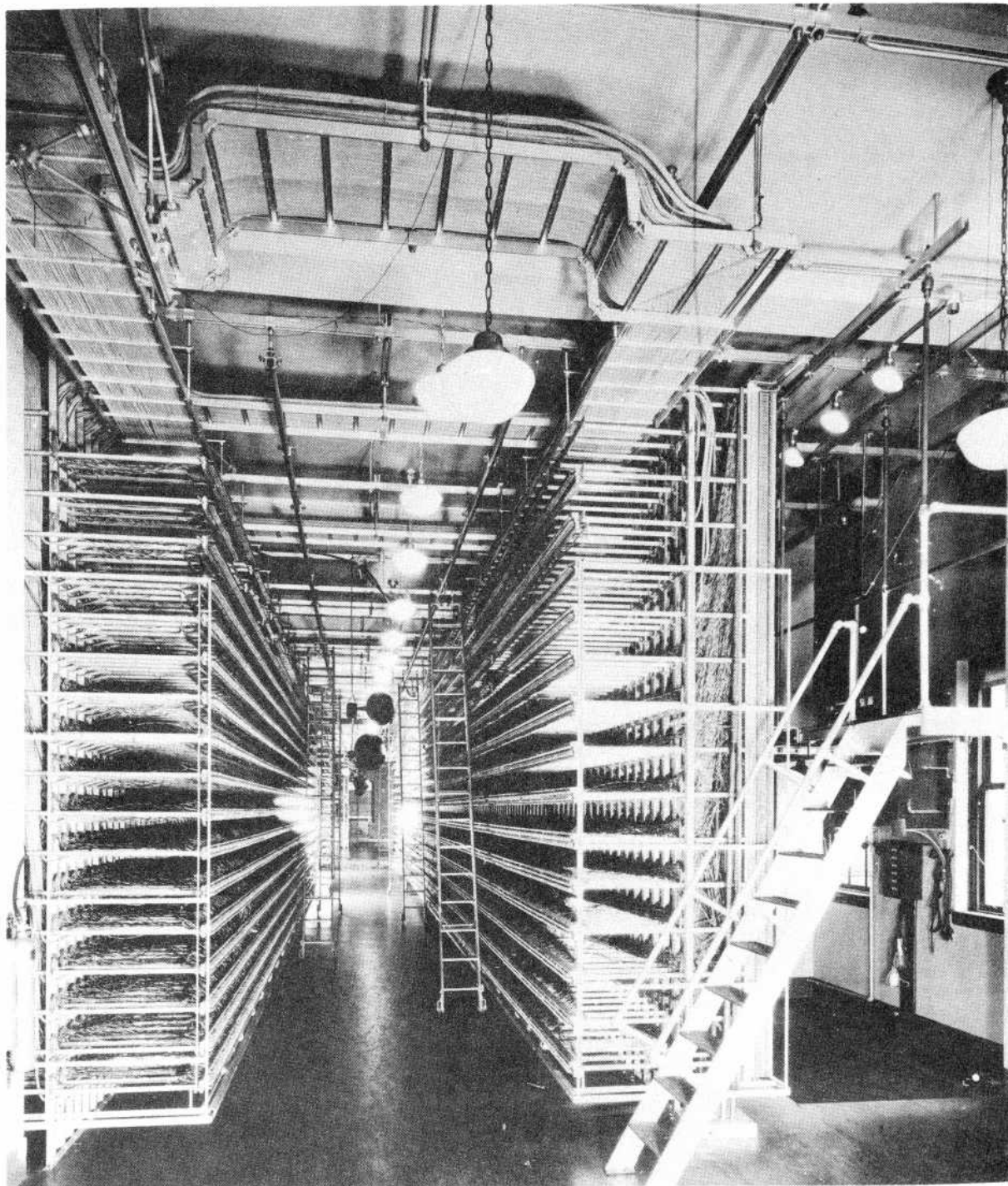
Figure 31 - Main and Intermediate Distributing Frames
