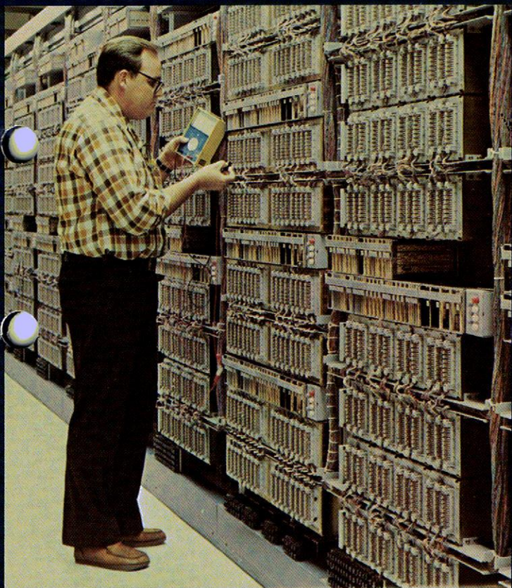
Testing Line Link Frames
