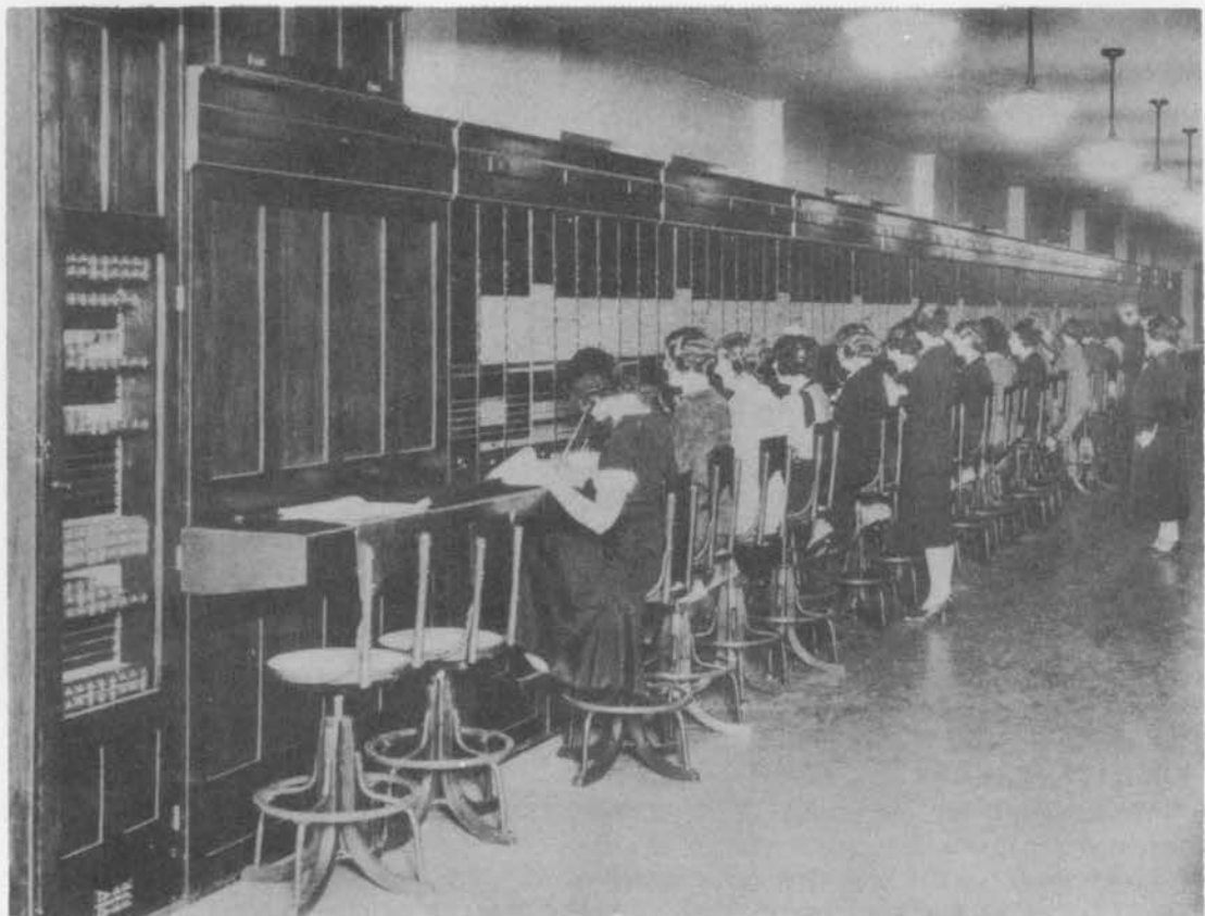
Fig. 9 606A PBX Switchboard
