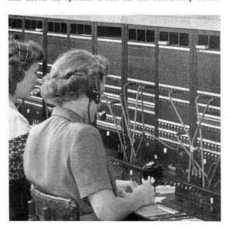
floor. Keyboards are extra wide with removable glass bulletin holders. Each keyboard is arranged for mounting both a dial and a key sender set. It has a capacity of fourteen cord circuits, with common keys for splitting, coin control, dial, "wipe out" and "send rear."
