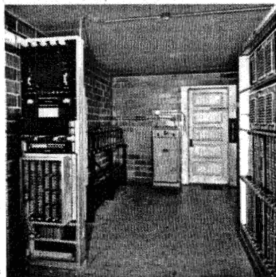
In this case the power panel is mounted alongside the main frame. A Leich vibrator type ringing converter is mounted on the back of the panel. A battery charger, floor mounted is near the door. At the bottom of the power panel is an auxiliary relay bar frame for mounting miscellaneous relay bars.
