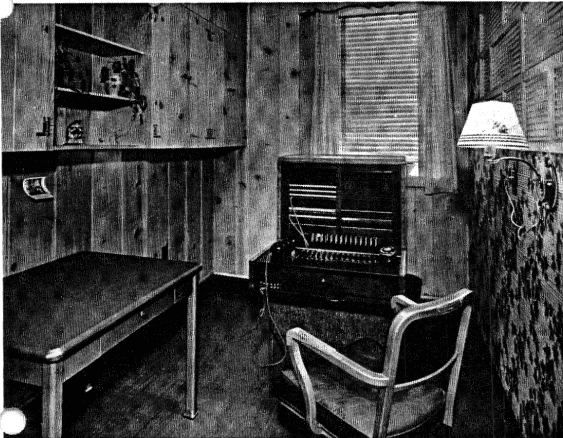
Leich attendant's cabinet for Leich Dial System PABX at the Michigan Consolidated Gas Company in Muskegon.
