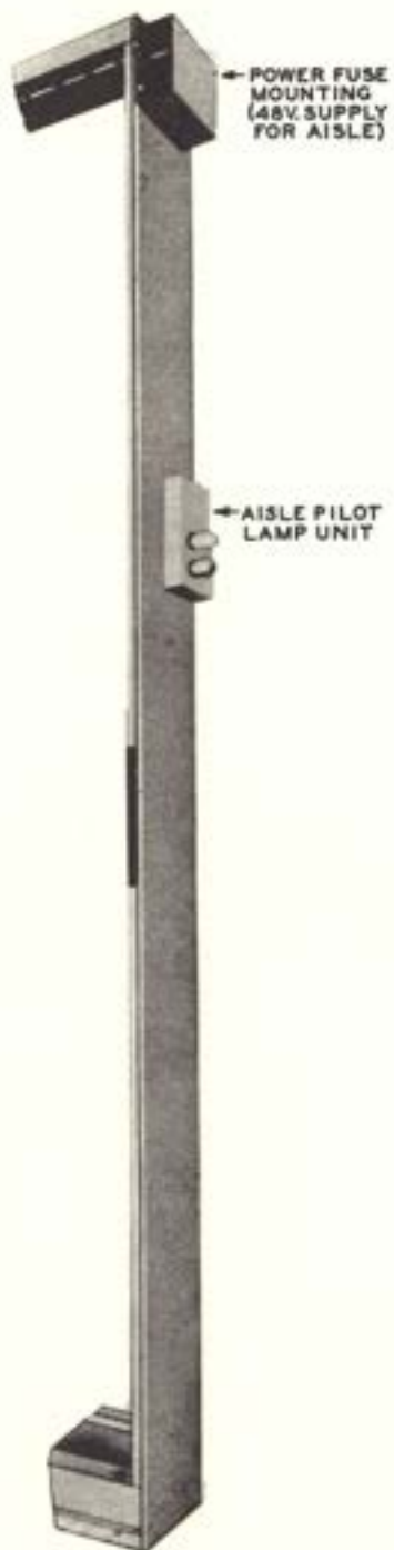
END GUARD WITH AISLE FEEDER FUSES AND AISLE PILOT
