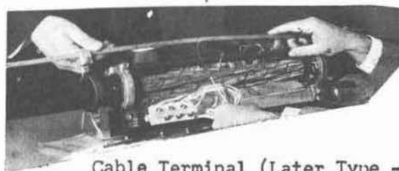
Cable Terminal (Later Type - Mounted on Cable instead of Pole.)
