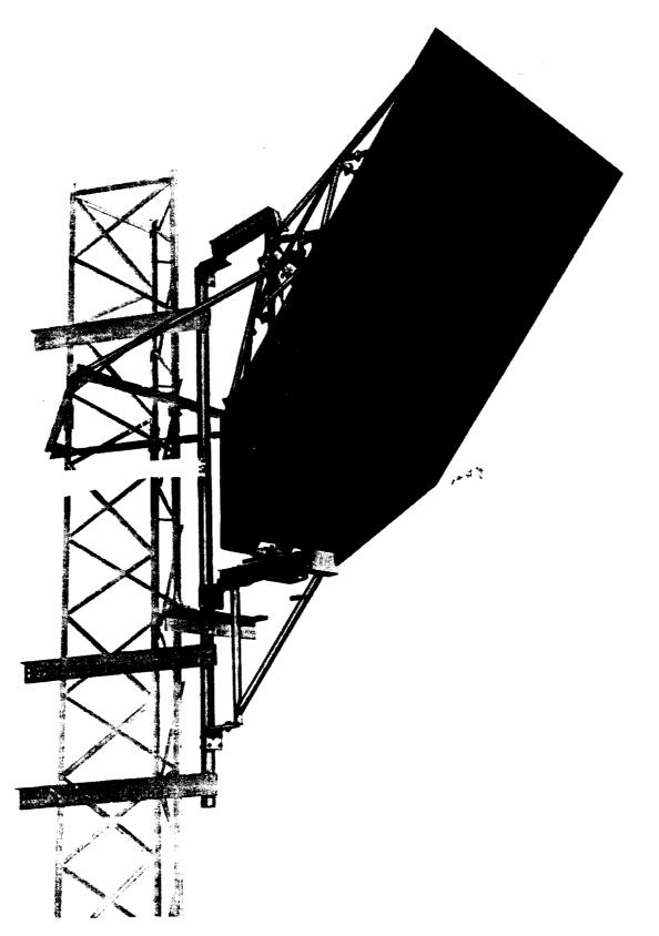
Fig. 1 — Typical Passive Reflector — Front View
