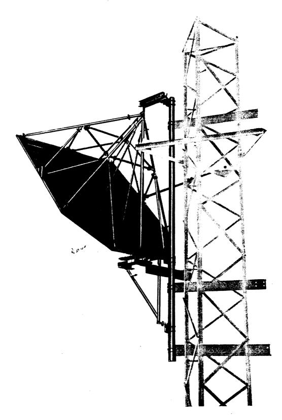
Fig. 2 — Typical Passive Reflector — Back View
