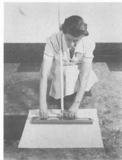
Fig. 2 – Rest handle on shoulder. With both hands free, tuck near edge of cloth under lip of the boot. Outer sides of cloth pass through slot in each corner of boot to overlap tool on each side. Tuck cloth well into slots in corners of boot.
