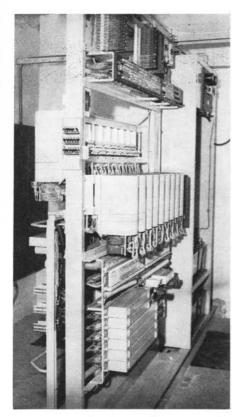
Front view of a line frame and its power supply.
