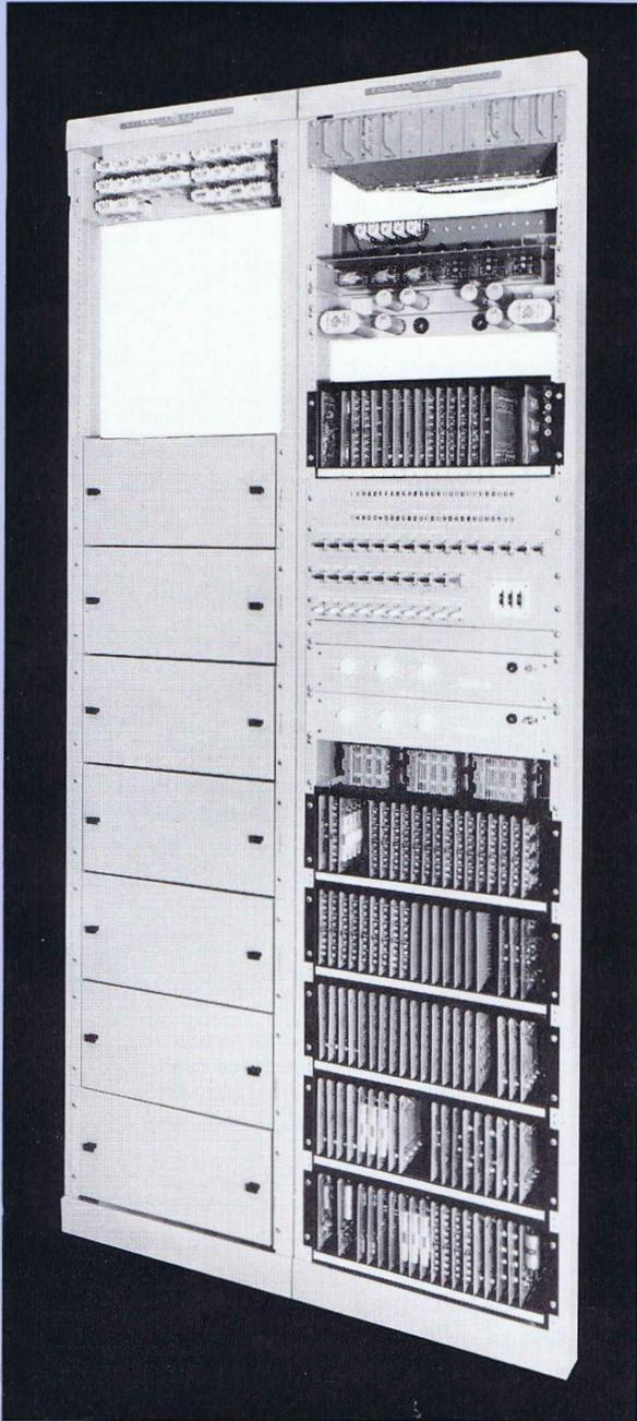
Figure 4. Master-station equipment is mounted on open-relay-racks—tone and line switching equipment at the top, maintenance panel and digital clock and calendar at the center, and system control logic and buffer storage for the teletypewriter at bottom.
