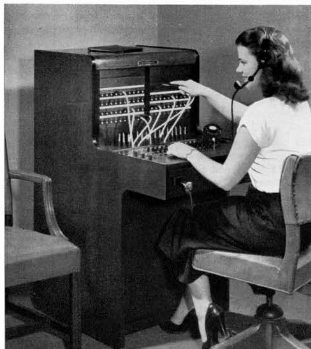
The No. 128 PBX Switchboard
