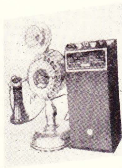
The 1907 model desk telephone adapted to paystation use with the coin box attachment for nickels, dimes and quarters.
