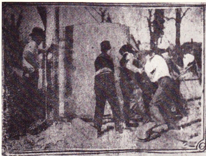
Unusual picture of an Automatic telephone sub-office, installed in Columbus, Ohio, about 1906. The board was sunk below ground in a vault. One of the earliest "unattended" exchanges.
