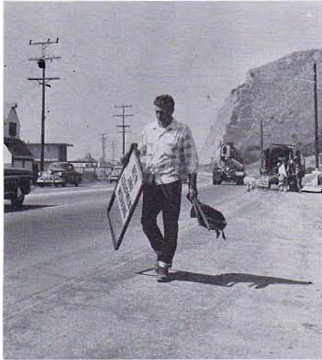
An important step — placing warning signs before starting the job. Below, on Coast Highway near Malibu, Bill helps crew load trailer to truck after placing underground cable.
