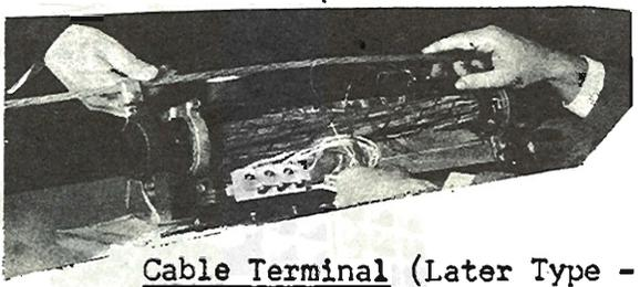
Cable Terminal (Later Type - Mounted on Cable instead of Pole.)
