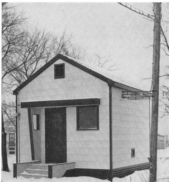
Figure 2. Exterior view of Warren office, showing original design of prefabricated building and aerial cable entrance.
