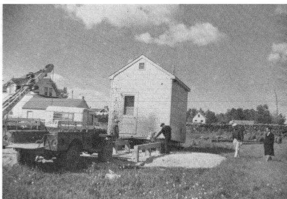
Figure 10. Building being hauled on to foundation beams by power winch.
