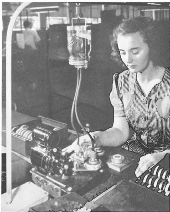
Not a blood transfusion, but a new device for replacing carbon crystals in telephone transmitters
