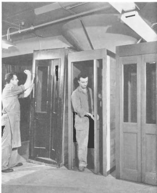
Telephone booths which bear the marks of hard use are scraped clean of their scars and made fit for more years of service
