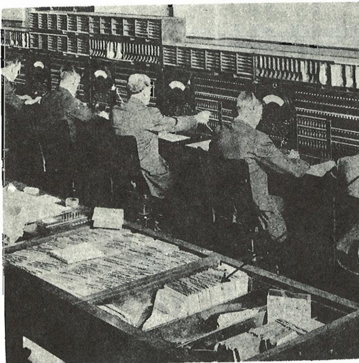
← LTD - Local Test Desk, for checking outside Subscriber Lines and Trunks that are in trouble.
