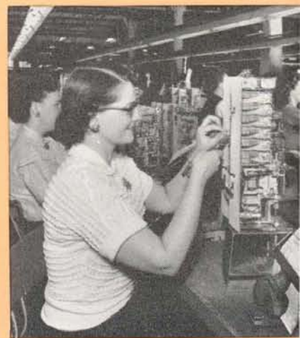
Wiring Strowger switch base
