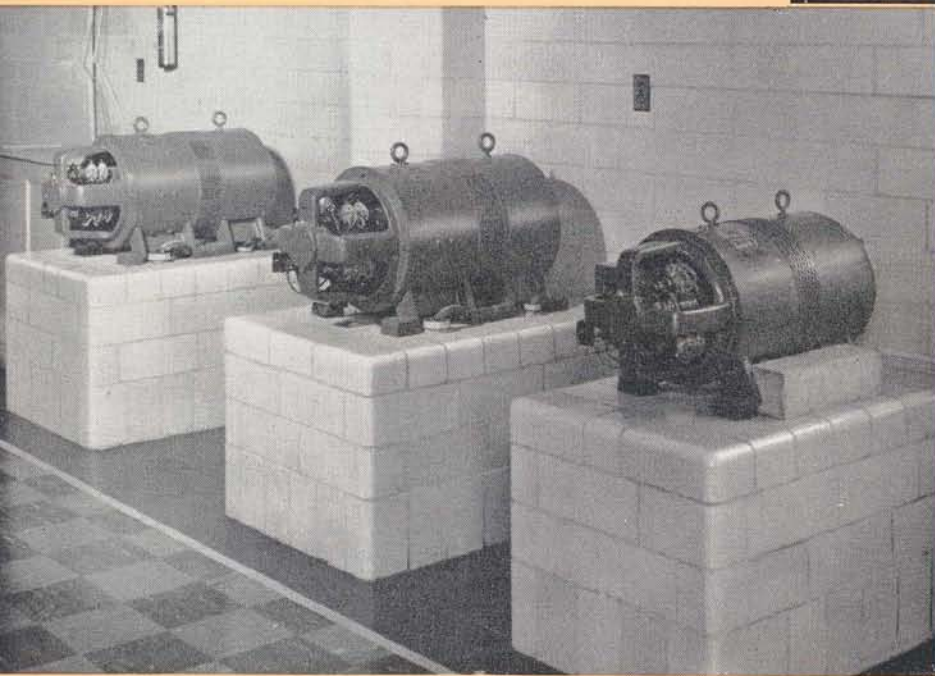
Motor-generators as used in a large Strowger Automatic Exchange.
