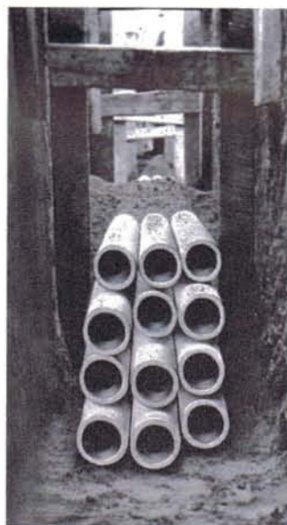
Transite Duct Are Installed in Direct Contact, Saving Trenching Time and Backfilling.
