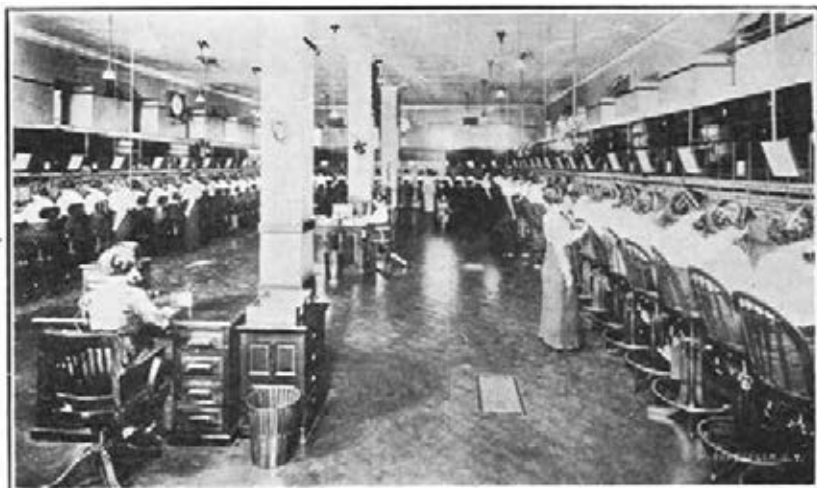
View of Multiple Switchboard in Chelsea Office, New York City, Cut in Over Eighteen Years Ago and Still in Operation.
