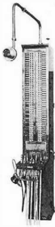
View of 41 Wire 4 Jack Toll Test Board
