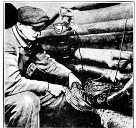
Solder joins the wires in lead covered cables and also joins the lead sheaths where two cables come together, thus preventing moisture from creeping in to injure the insulation.
