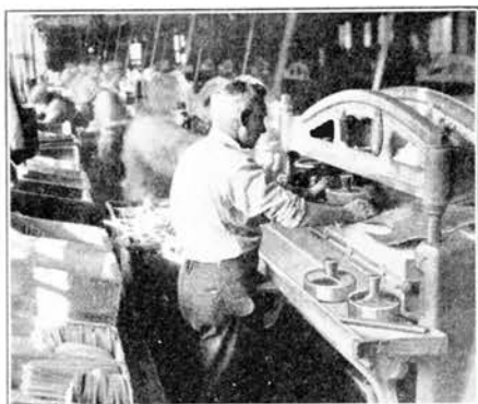
A die cutting machine, making blanks for the base of telephone handsets.
