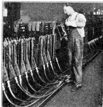
Asphalt in cable terminals, used when telephone wires are joined to a lead covered cable, prevents moisture working in among the wires.
