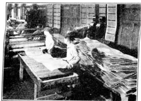
Straightening sheets of aluminum by rolling them.
