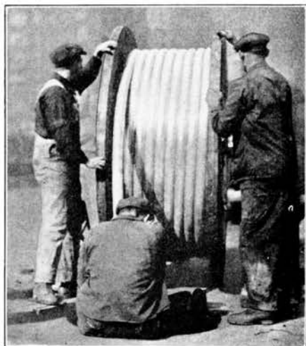
In this familiar scene the telephone wires are being put underground, enclosed in their protective sheath of lead.
