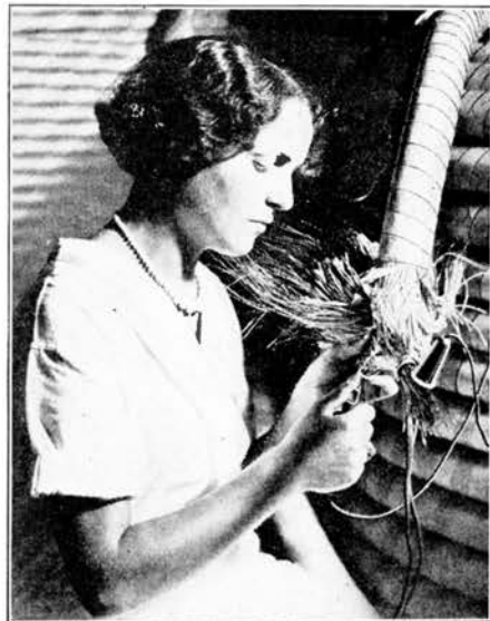
This shows the paper wrapped wires in a cable and the paper wrapping around the entire rope-like group of wires, just as the cable core looks before it receives its sheath of lead and becomes real lead covered cable.
