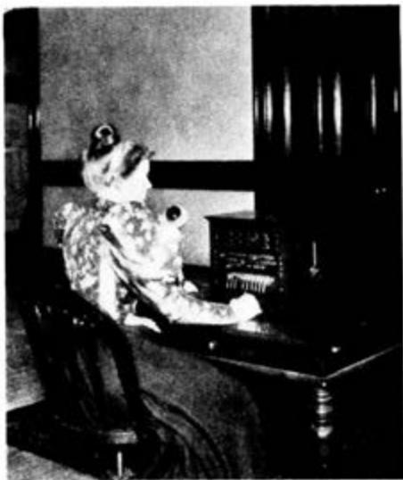
Fig. 6-96. PBX switchboard for ten or less telephones. (From Electrical Engineer , November 25, 1897)
