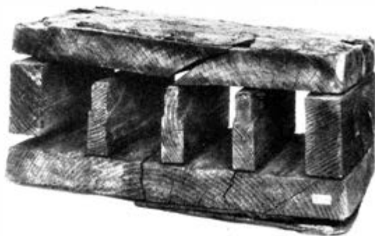
Fig. 4-20. Early creosoted wooden conduit.
