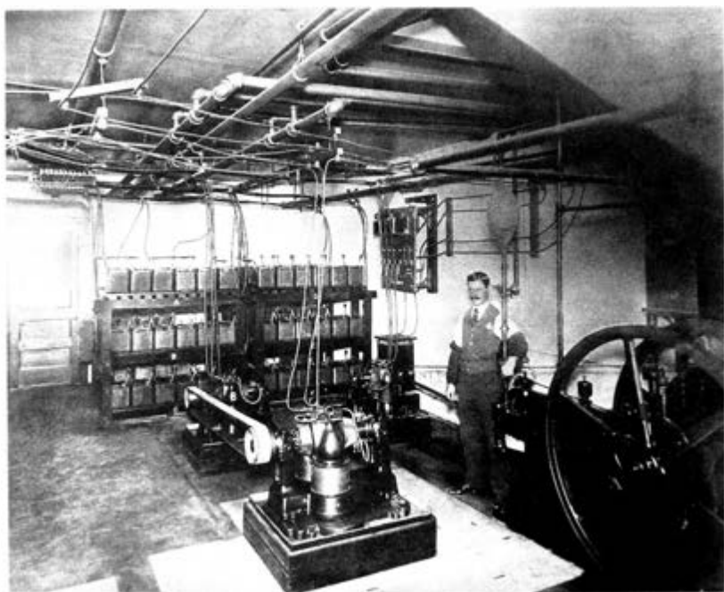
Fig. 6-119. Power plant in Worcester, Massachusetts, common-battery office, 1896.
