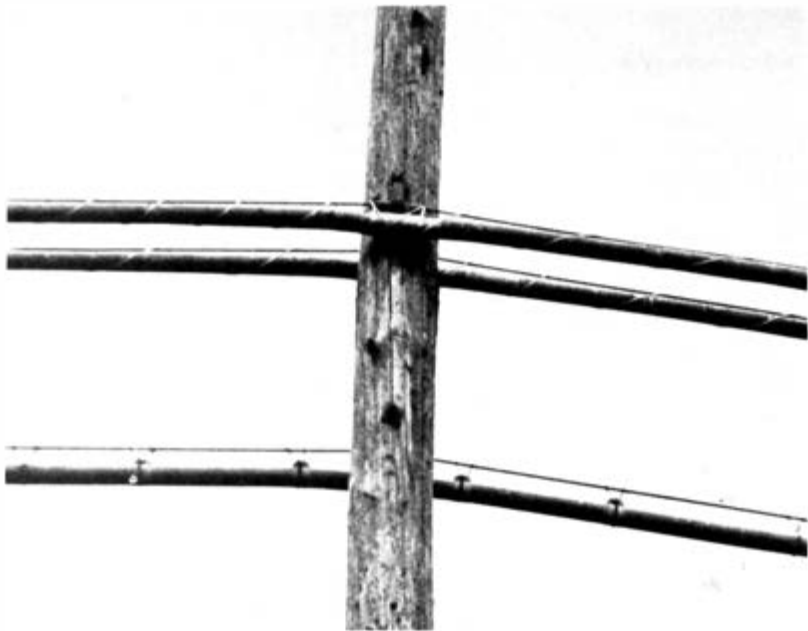
Fig. 4-15. Cable supported by wire "messenger." Wire hangers support lower cable; lashing is used on upper cables.
