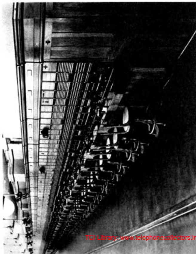
Fig. 6-82. No. 3 toll switchboard, Chicago, 3,400 lines.
