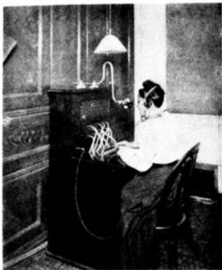
Fig. 6-95. Large PBX switchboard at the H. B. Claflin Company, New York City. (From Electrical Engineer , November 25, 1897)
