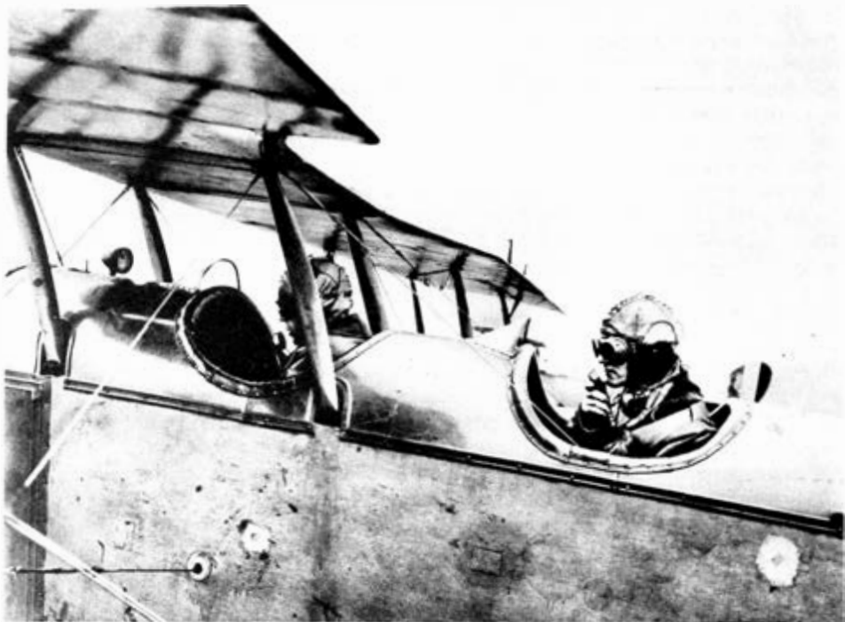
Fig. 5-17. Telephone receiving helmet for airplane radio. (Craft and Colpitts 1919, Fig. 40)
