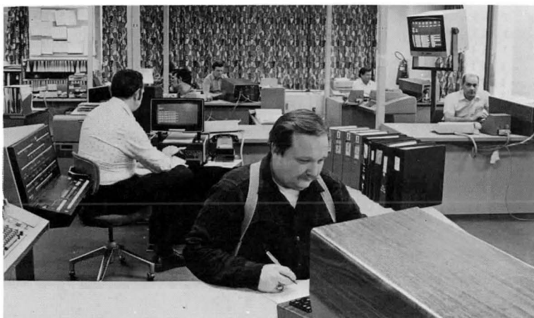
Figure 15-3. A typical Switching Control Center. One of New York Telephone's Switching Control Centers is the hub of local switching office surveillance, testing, and maintenance for over a dozen central offices. Switching equipment technicians are assisted in their work by computer-based operations systems.
