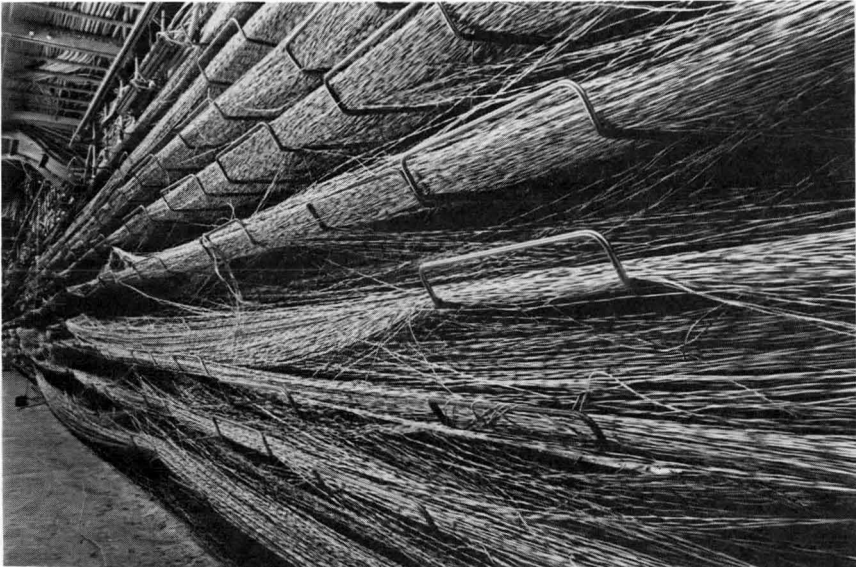
Figure 12-10. An overloaded main distributing frame in a central office.
