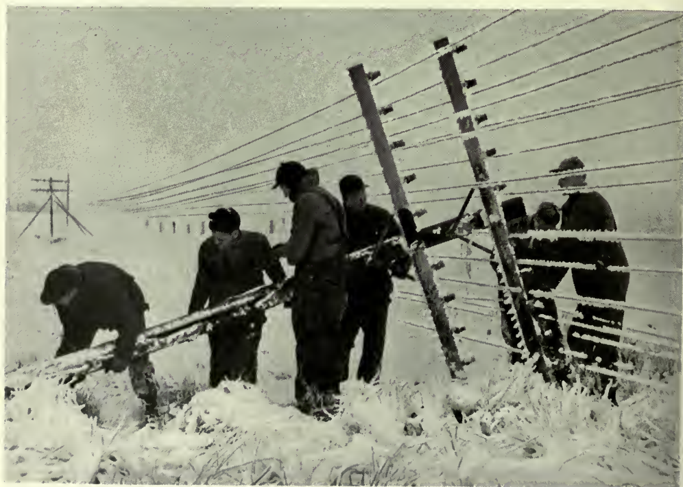
Lines of the Indiana Bell Telephone Company (above) and the Illinois Bell Telephone Company were victims of the New Year's sleet
