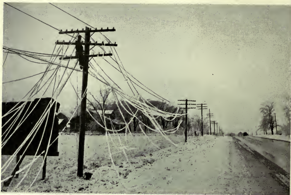
Lines of the Indiana Bell Telephone Company (above) and the Illinois Bell Telephone Company were victims of the New Year's sleet
