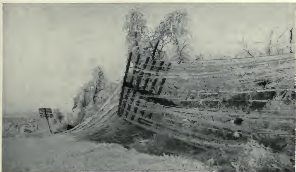
What the sleet did to this Dallas-St. Louis line near the Texas-Oklahoma border is typical of the destruction over a wide area
