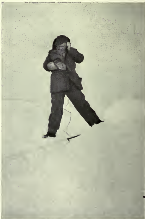
To clear a case of trouble here, this combinationman had to dig down to the wires on top of 20-foot poles
