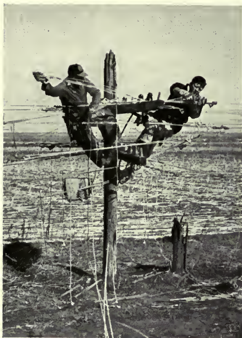
Temporary restoration near Abilene, Tex.: a broken pole reset to get the toll lead back into service
