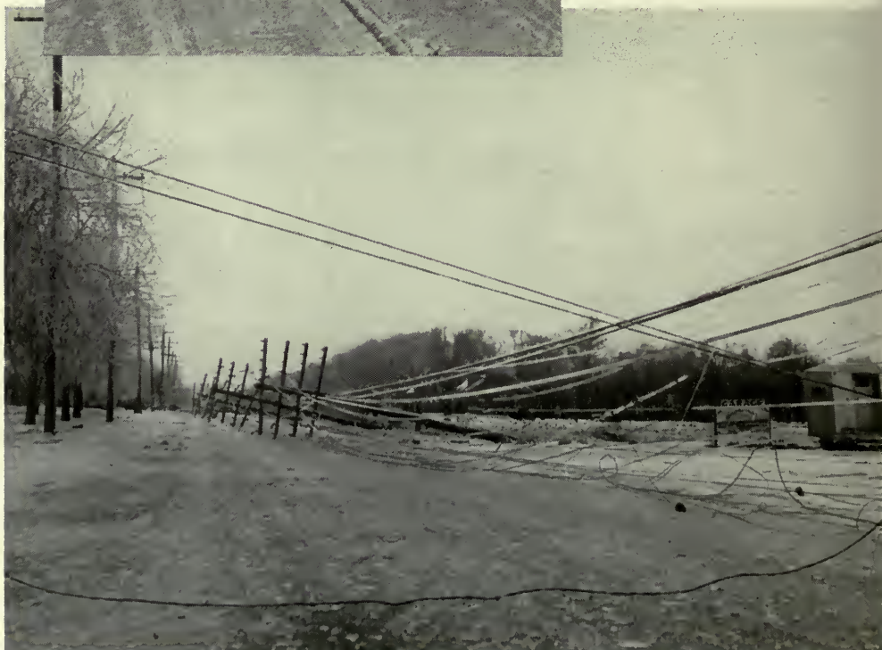
The January 1 sleet storm invaded the territory of the Bell Telephone Company of Canada to fell a pole line on the outskirts of Windsor
