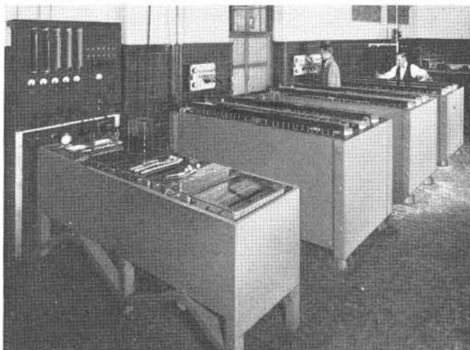
*Fig. 5—In the plating room, of which G. E. Wenzel (right) is foreman, current for the large plating baths is controlled from individual switchboards, at one of which is A. B. Celner. Current for the smaller baths is controlled at the switchboard in the foreground*
