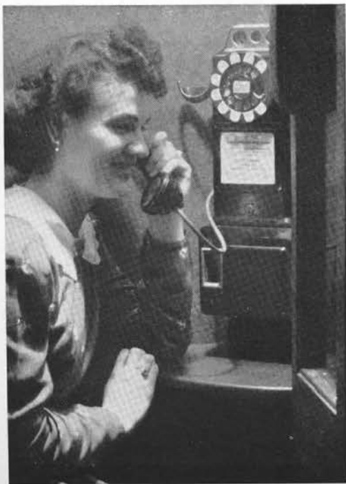
Fig. 1—Substitute materials save approximately 85 pounds of steel, 25 of rubber compound, and 10 of brass and bronze in the construction of the wartime telephone booth
