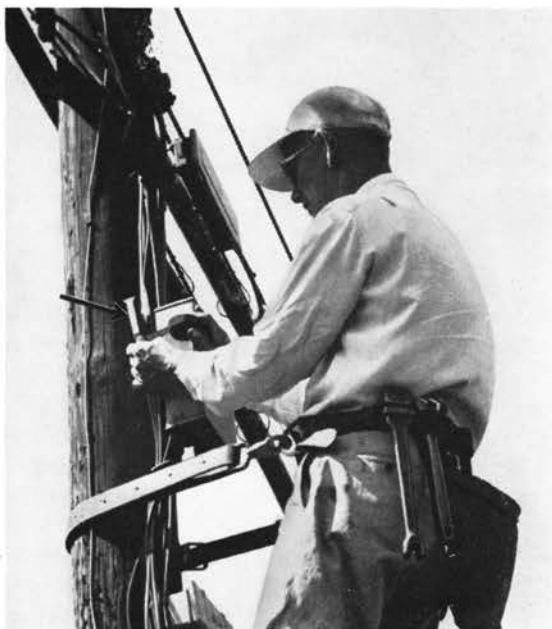
T. W. Rolph places B Drop Wire Cap (arrow) on disconnected wire.
