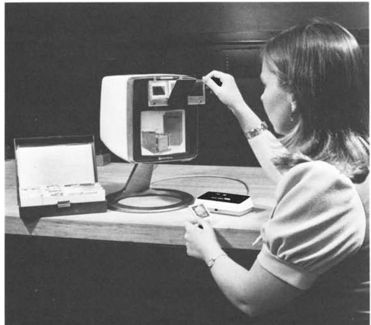
*A clear plastic holder and a close-up lens allow the viewer to send images of 35-millimeter slides. A reflector at an angle throws ceiling light on the slide—additional light is not needed.*
