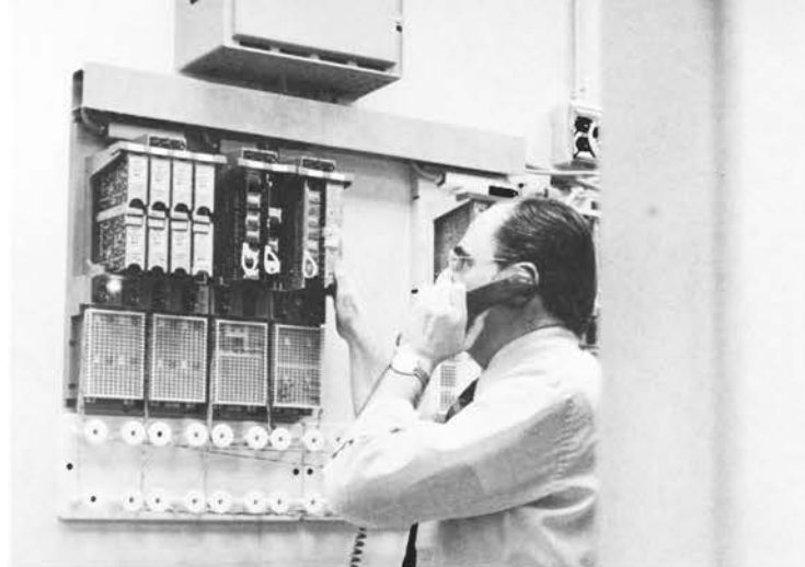
At the Holmdel, N. J., location, Bell Labs engineer Robert McAlonie adjusts the dial tone on a new 1A2 key telephone system with modular panels. This installation is used by the Bell Labs Customer Telephone Systems Department, which is responsible for development of the 1A2 and its peripheral equipment.
