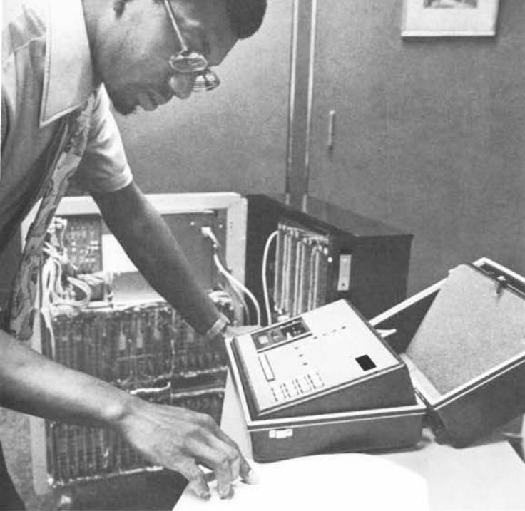
**Easy access.** Taking advantage of stored program control, Bell Labs engineer Harold Woodland uses a portable Service Access Unit to change a *HORIZON* System's line arrangements.
