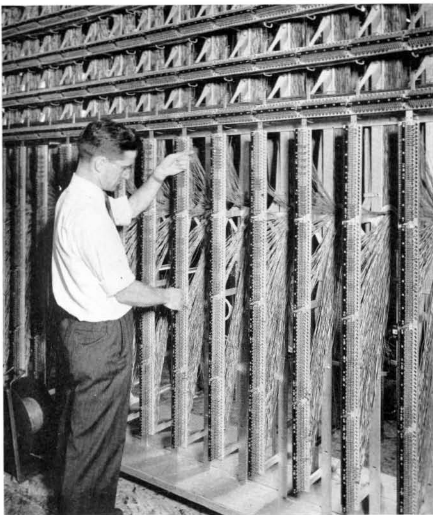
Assignment distribution frame for crossbar toll
