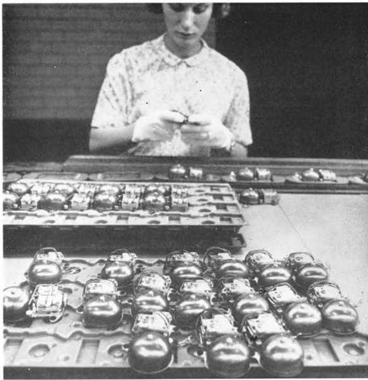
Each ringer is carefully adjusted during manufacture at Indianapolis. These M1A ringers will be used in Princess telephones.
