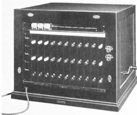
Fig. 1—Outer view of the 506-A switchboard. The other three pictures also show this switchboard
