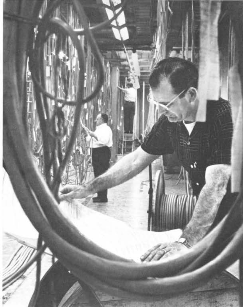
Crewmen working on a CENTREX exchange being installed for the New York Telephone Company.
