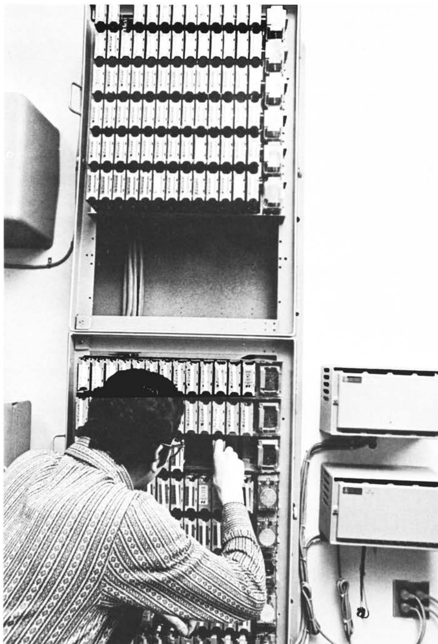
The cabinet, which houses the key telephone circuit equipment for the Newark, N. J., office building, is located in the same room as the wiring facility with the circuit terminals.
