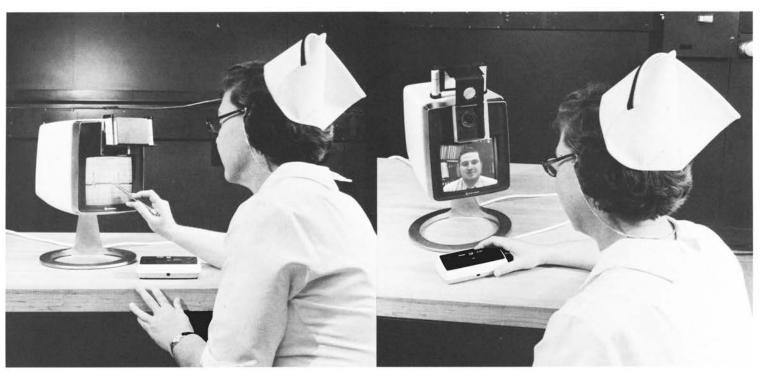
With the electrocardiogram reader, an EKG record can be transmitted to a medical expert at a remote location (left). The reader consists of a close-up lens and a support that keeps the chart in
