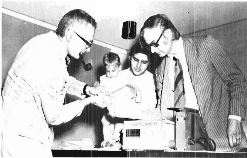
Fig. 6-18. The portable testing device for lead poisoning developed by Bell Labs scientists, shown being demonstrated at a Massachusetts Governor's Conference on childhood lead paint poisoning. Dr. R. Klein, left, director of the state's childhood lead poisoning prevention program, tests an infant while her father and Bell Labs' W. E. Blumberg, right, one of the developers of the testing equipment, look on.
