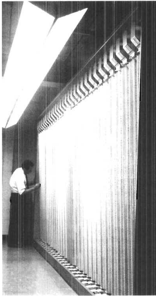
Fig. 11-38. Main distributing frame for No. 1 ESS, requiring one half or less of the space required for earlier MDFs.
