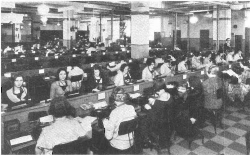
Fig. 13-70. Western Union installation of No. 3 order turrets, developed in 1932. The No. 3 was the first turret with automatic call distributing and call sequencing.
