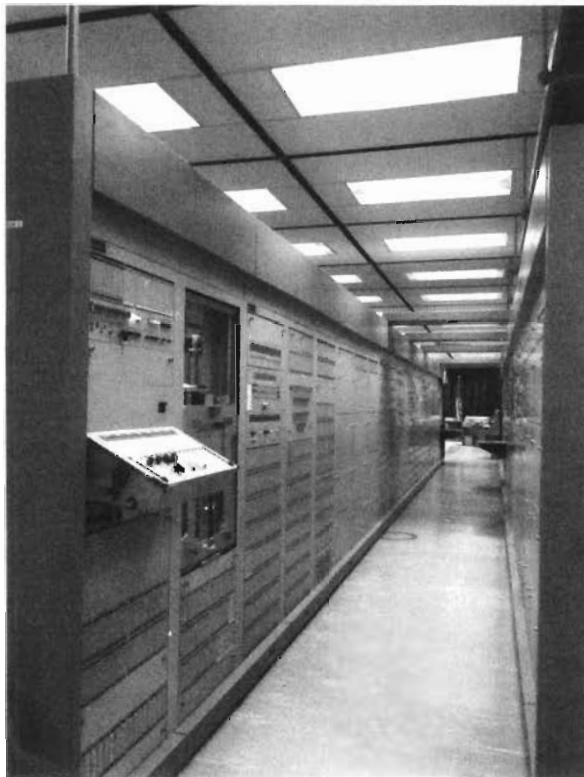
Fig. 9-47. Row of UNICOM switching equipment which employed forced air cooling, an example of special design to meet military requirements.
