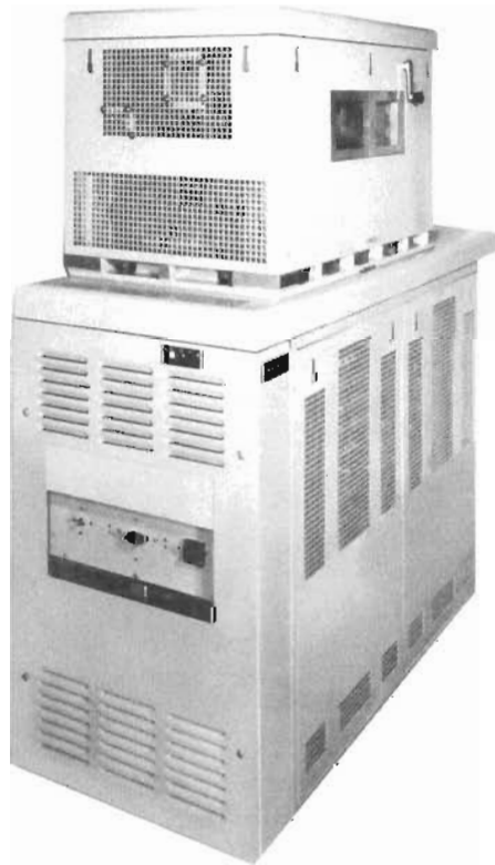
Fig. 8-6. A card translator, a development that filled the need to receive 10 digits and translate 6. The card translator speeded nationwide direct distance dialing.
