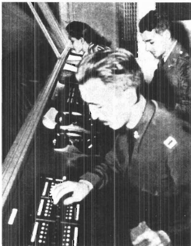
Fig. 13-83. Wartime personnel using 101-type key equipment to communicate information derived from air raid observers.
