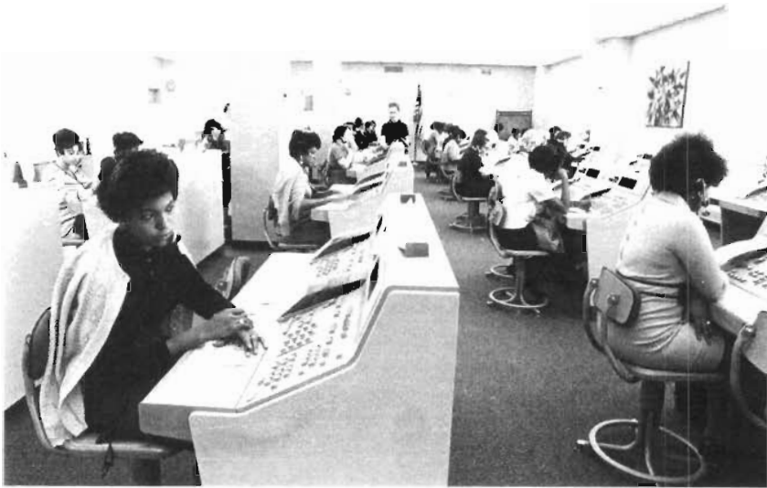
Fig. 10-7. Traffic service positions, with their desk-like consoles, allowed a more attractive environment for operators.
