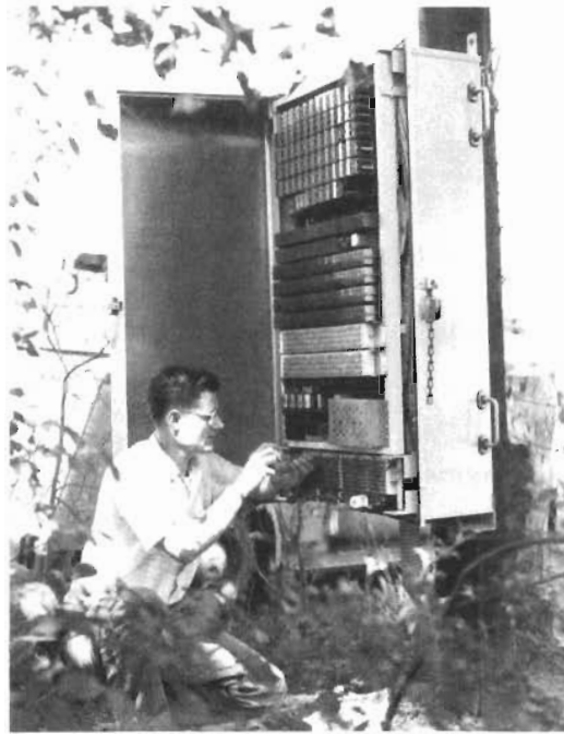
Fig. 11-35. Pole-mounted 1A concentrator unit. Magnetic-latching crossbar switches reduced power requirements.
