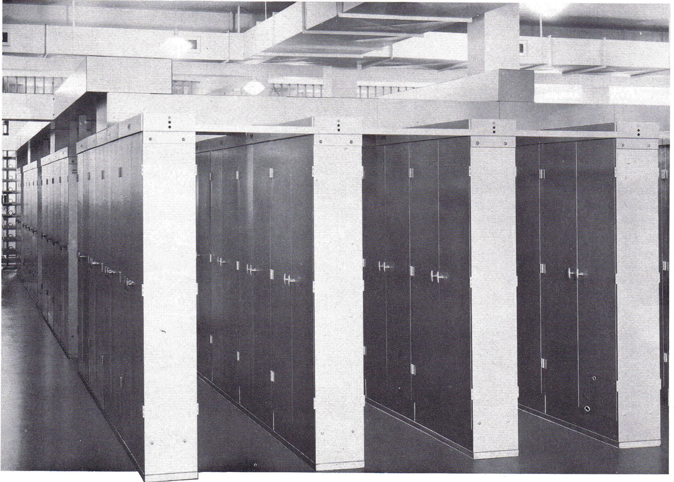
Typical installation of a North All-Relay CX 10,000 exchange initially equipped with 1,000 lines.
