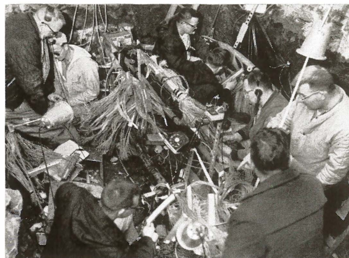
A line crew in the cable pit, painstakingly splicing thousands of wires in one cable to their mates in another.
