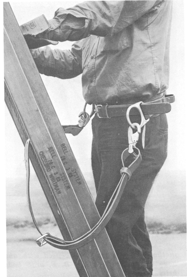
Fig. 7—Method of Using Safety Strap When Working From Ladder
