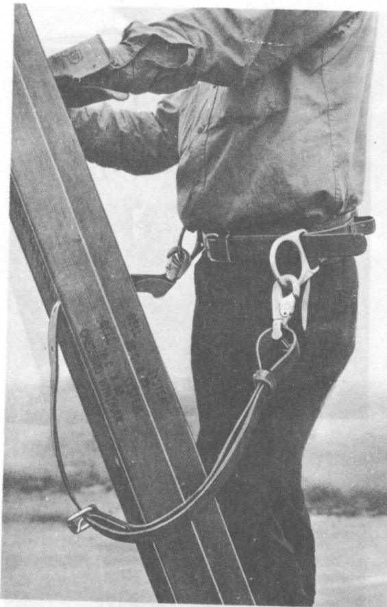
Fig. 6—Method of Using Safety Strap When Working From Ladder
