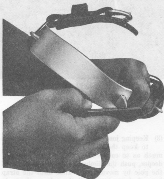
Fig. 17—Removing Burrs From Top Cutting Edge
