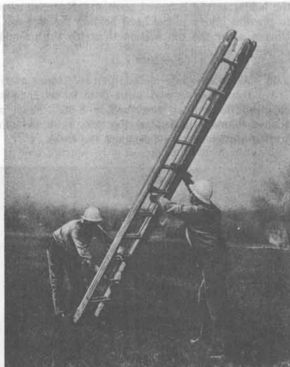
Fig. 26—Two Men Raising Ladder
