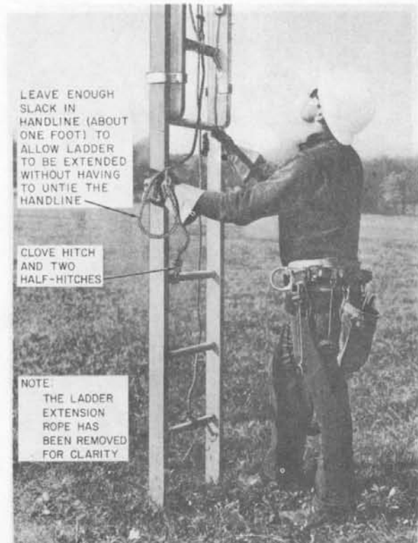
Fig. 23—Method of Securing Handline
