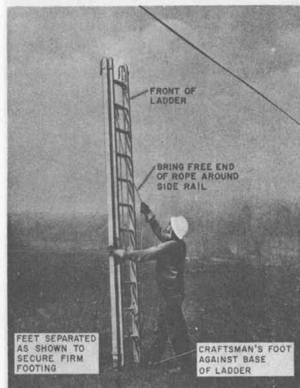
Fig. 27—Preparing to Extend Top Section
