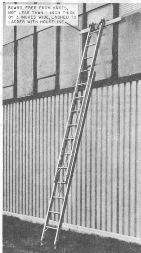
Fig. 10—Ladder Placed in Front of Window
