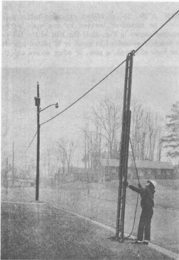
Fig. 22—Ladder in Vertical Position
