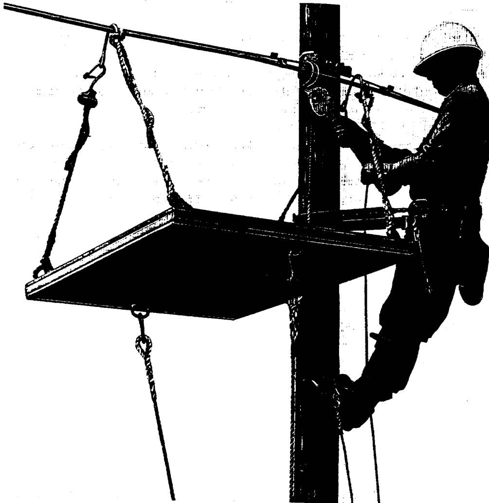
Fig. 9-E Platform Suspended at Pole
