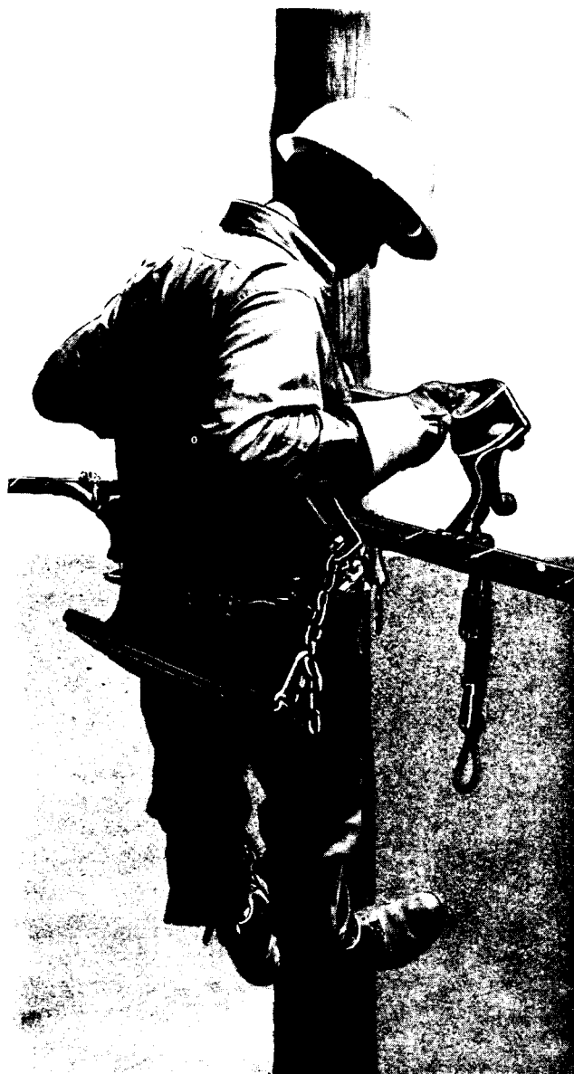
Fig. 9—Placing Car on Strand
