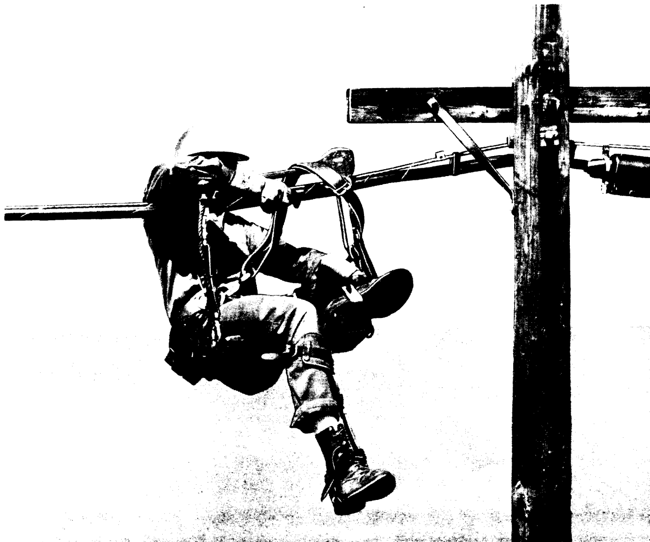
Fig. 7—Final Positioning in Cable Car Seat
