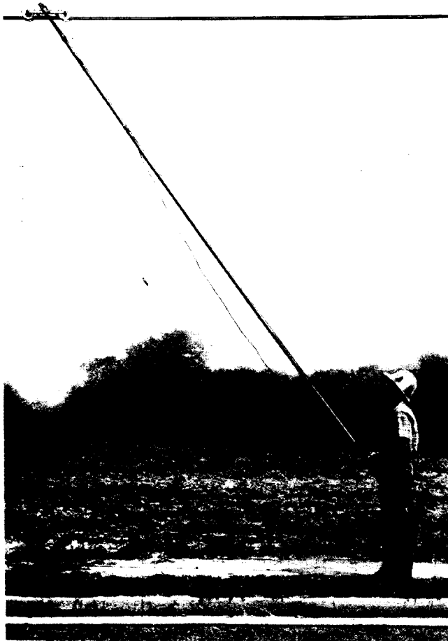
Fig. 18—Locating a Leak Using Trolley Method
