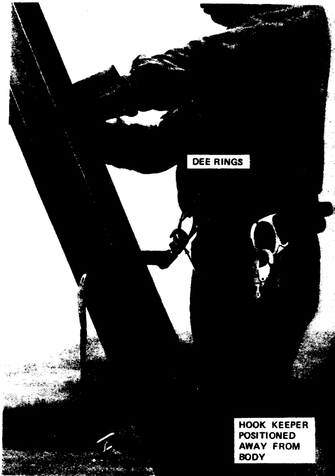
Fig. 4—Method of Using Safety Strap When Working From Ladder
