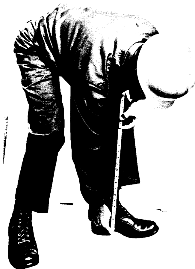
Fig. 9—Measuring for Climber Length
